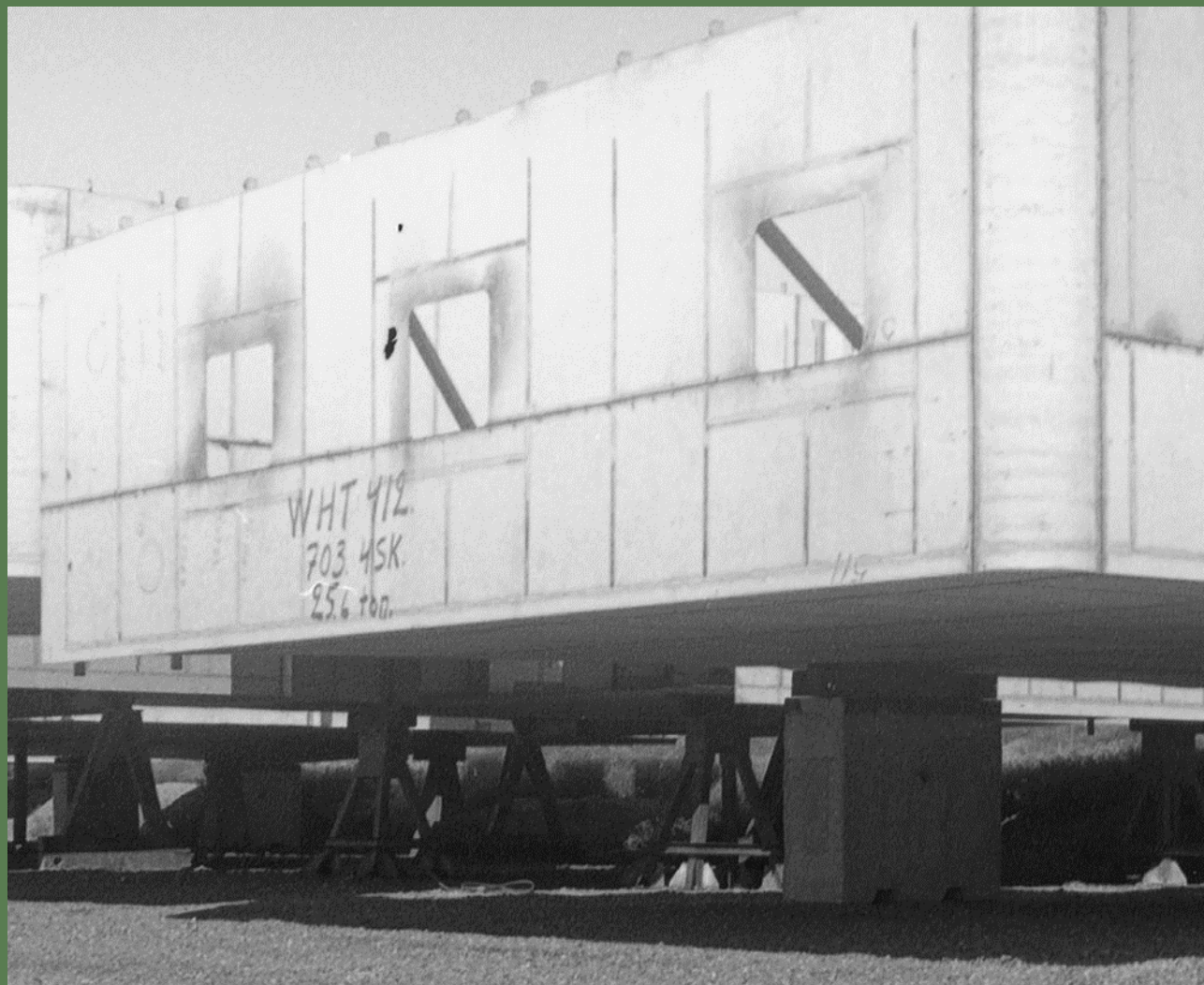
Segments of the Polar icebreaker Kapitan Nikolai under construction at the Helsinki Shipyard. Ship was delivered to Soviet Union in 1978. Teuvo Kanerva, latest 1978. (HK19950323:5765)
